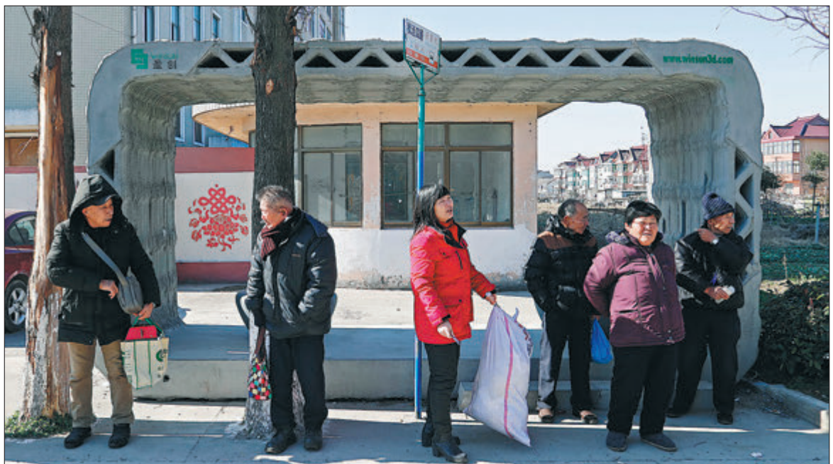
Shanghai has installed a set of 3-D printed bus shelters — believed to be the world's first — to serve a bus line in its suburban Jinshan district. The bus shelters feature a closed-loop design that looks like a rectangular frame measuring 16.7 feet long, 4.9 feet wide and 8.8 feet high. "All the printing materials are from recycled and classified industrial waste or tailings," said Wang Aijuan, who is responsible for the project at WinSun Construction Technologies.
